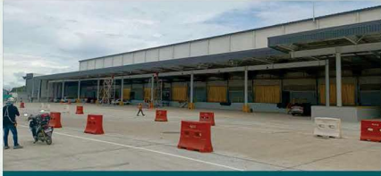
The Mega DC will feature 75 loading docks across the facility.
