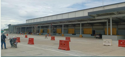
The Mega DC will feature 75 loading docks across the facility.
