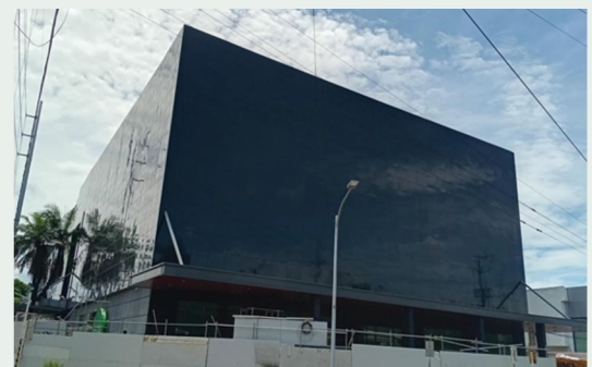
Green Sun Renovation Project
