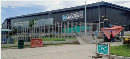
Progress Photos of the Facade of the Maersk Mega Dc
